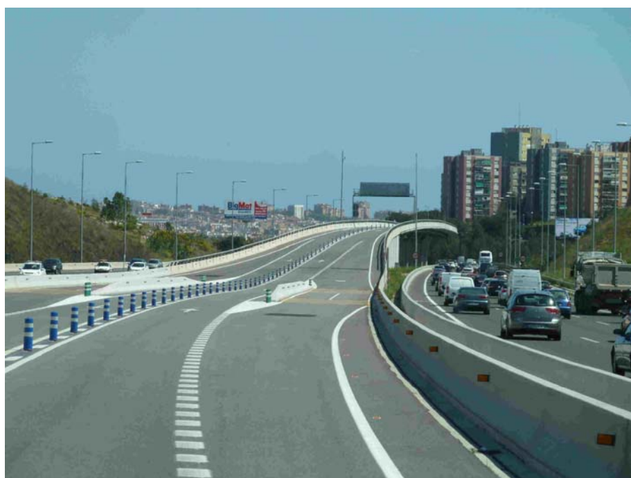
In the middle of the Bus-VAO section : by-pass at each side, for control operation by police
