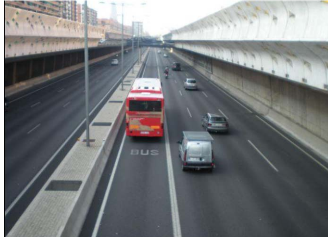
The bus lane (entrance of Barcelona), on the left is permanent No hard shoulder on the right
