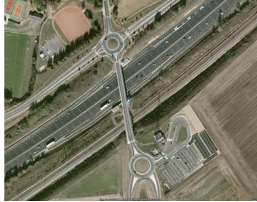
Aerial photo of the interchanges of Briis-sous-Forges.
