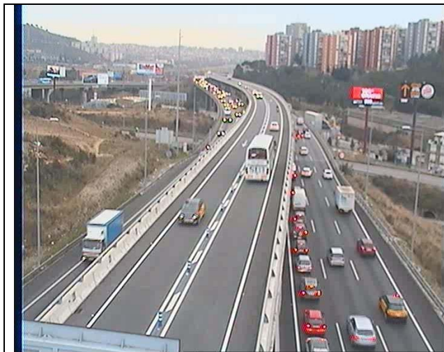
The 6,7 Km BUS-HOV with 2 lanes in the middle of C-58, on a separate road - The reversibility has been abandoned
