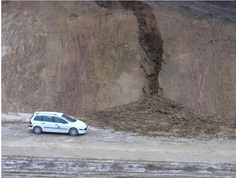
Figure 20: Erosion of a hillside in Brittany following heavy rainfall on 15 January 2008. Source: Olivier Malassingne (Cerema).
