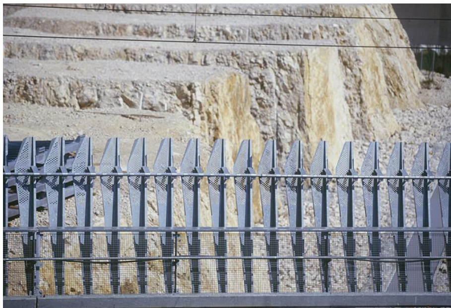
Figure 24: Deflectors on the Angles viaduct on the Mediterranean high-speed line. Source: SNCF Médiathèque, Jean-Jacques D'Angelo.
