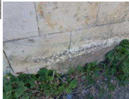
Efflorescences
