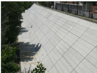
D12 Amidonniers : earthfill dike with concrete facing and piles
