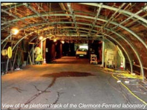
View of the platform track of the Clermont-Ferrand laboratory
